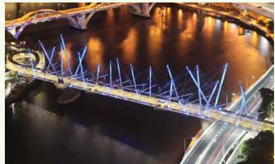
>Fig 2. Kurilpa Bridge Brisbane, Australia- World largest tensegrity bridge
