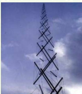
Construction: Iconic Needle Tower in Washington D.C, USA by Kenneth Snelson
